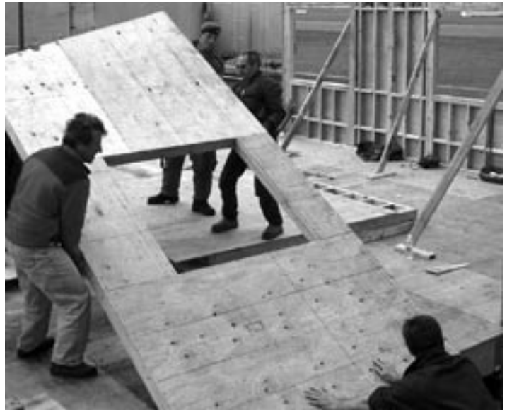
Lifting wall panel W5 into place.
