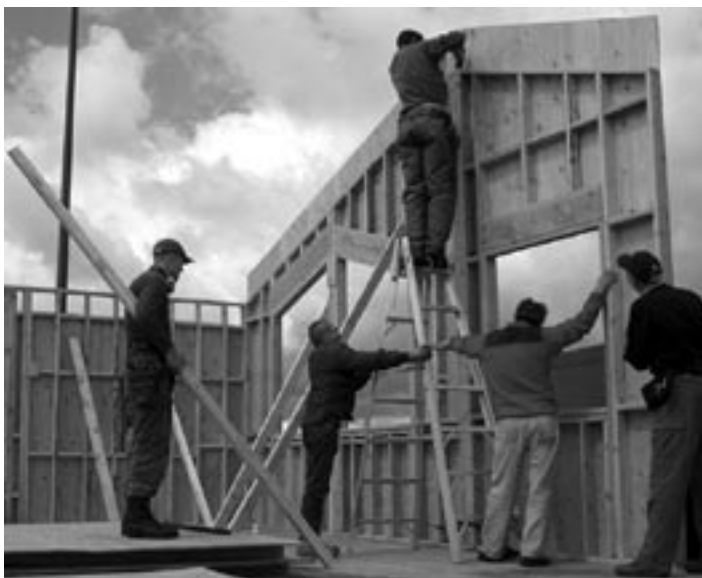
Careful alignment of the panels at the ridge, ready for bracing.
